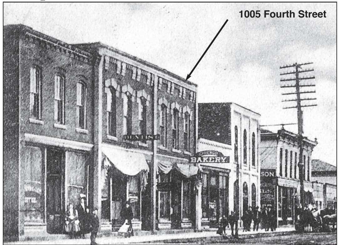
Pictured is the east side of the 1000 block of Fourth Street. 1005 is the third building on the left. 1003 and 1005 have the same outward appearance at the time of this photo. Photo circa early 1900s.
